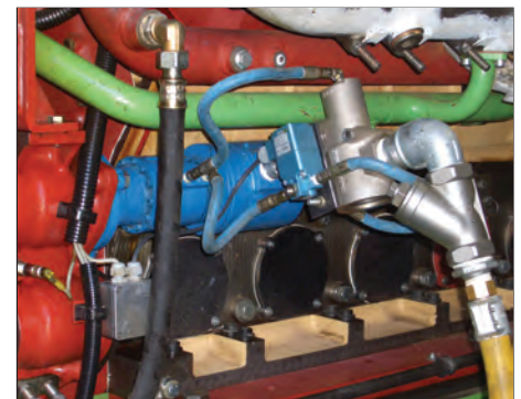
T30-Y installed on GE-Jenbacher GMD 312 engine.
