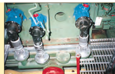
A trio of T100-Ds on a Clark gas engine provide the reliability to handle the higher cranking speeds.
