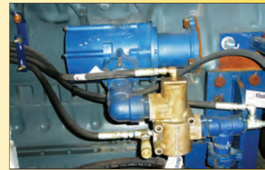
T100-F installed on Detroit Diesel 16V2000 engine.
