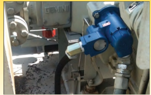
T20 on CAT G3306 compressor.
