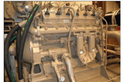
T106-F installed on Caterpillar 3412 engine.
