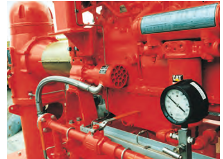
T306-I mounted on Caterpillar 3406 Engine for fire pump application
