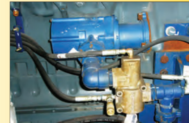
T100-F installed on Detroit Diesel 16V2000 engine.
