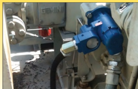
T20 on CAT G3306 compressor.
