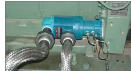
T50-P installed on Caterpillar 3516 engine.
