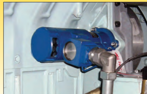
T25 installed on MAN D2842.
